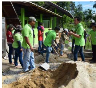
▶ STA – PL School ‘s Toilet improvement
